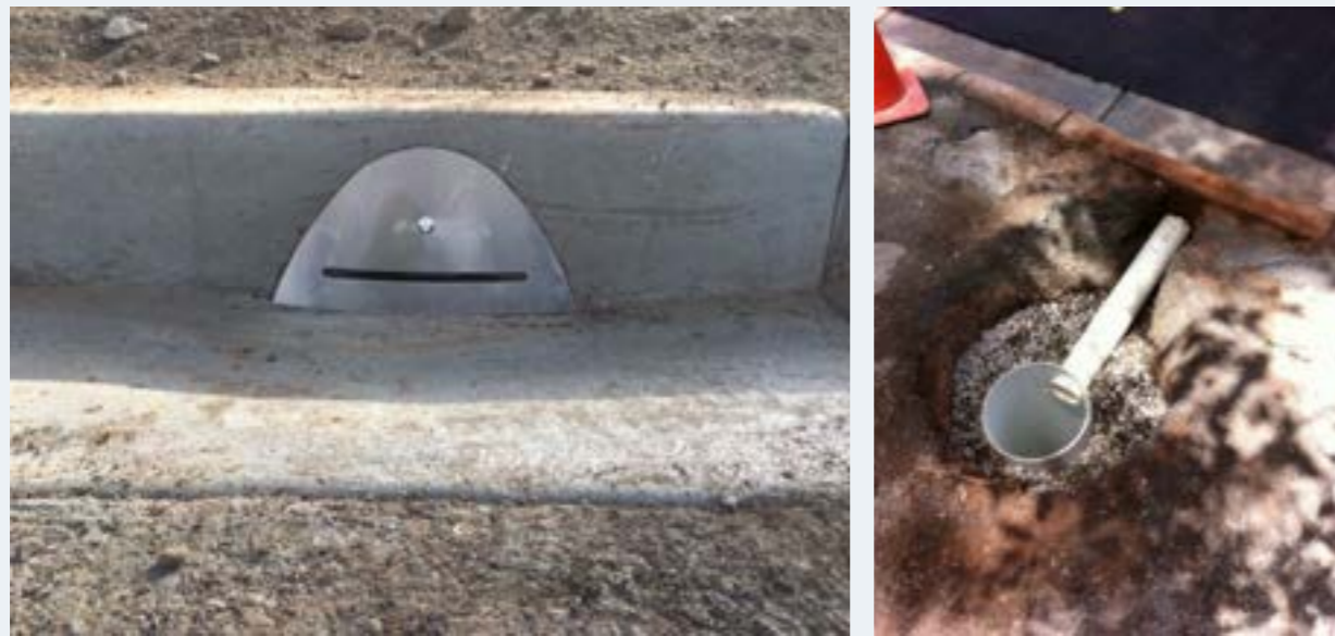
Above images: A TREENET Inlet (pictured above) designed by Space Down Under delivers water to the soil of the street verge (nature strip), providing added water supply for street trees (Johnson, 2022)
