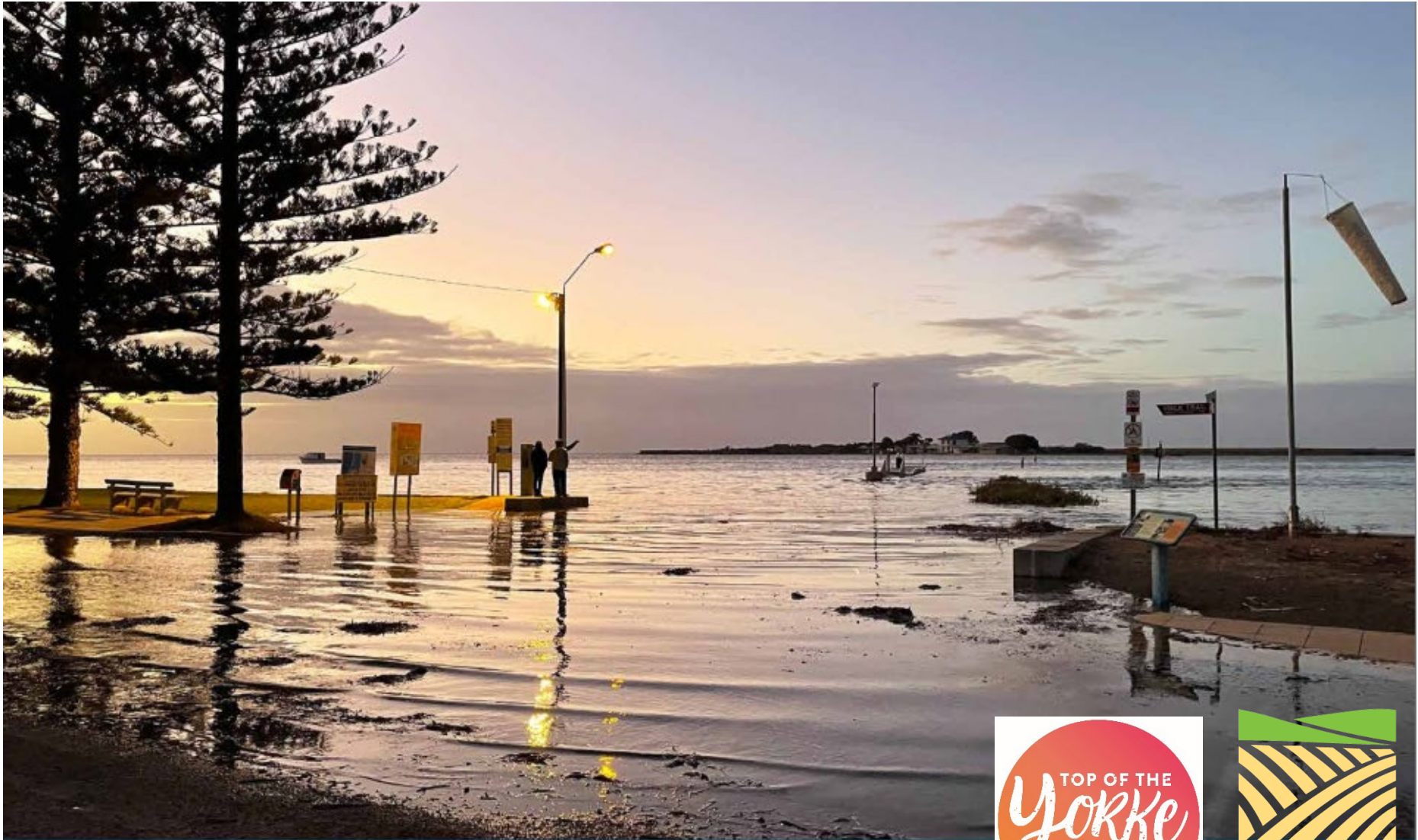
2016 FLOODS - FISHERMAN BAY BOAT RAMP
