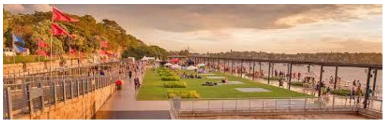
Figure 17: The Coal Loader Platform
